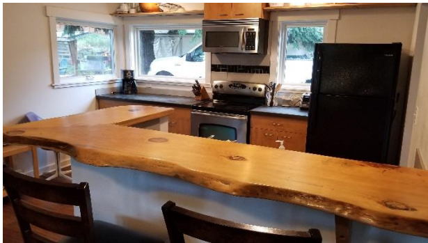
Morales Farmhouse After FotF Renovation
